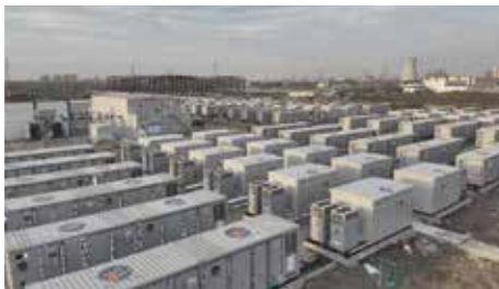
◆ Lianyungang Energy Group Independent and Shared New Energy Storage Project Location: Jiangsu Province, China Scale: 150MW/300MWh
